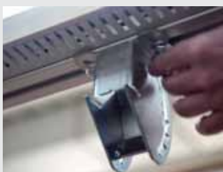
Step 1. Install the bracket
